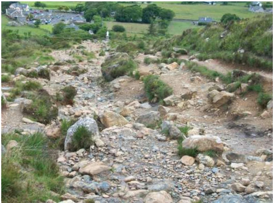
Section 1 – Looking northwards down the path to the start – braiding and turf “islands” very apparent, as is lack of any drainage. During heavy rain this would resemble a stream.
